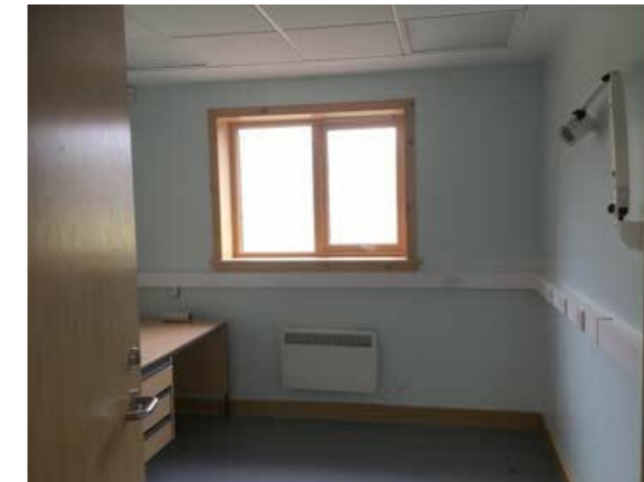
Former medical room to be converted to an ensuite
