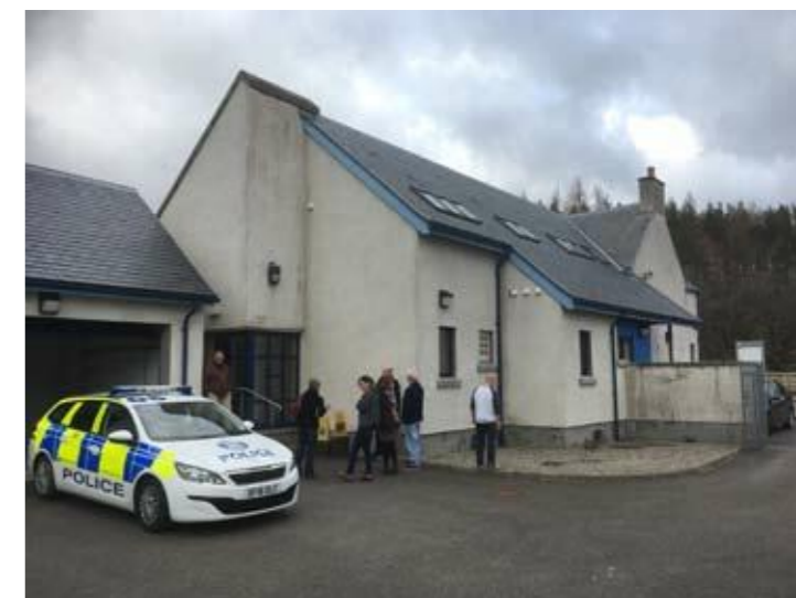
On site parking for 6 cars
