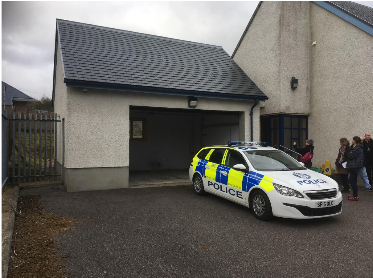
The garage at the Police Station, Lairg which could be used as a secure bike storage and drying area.
